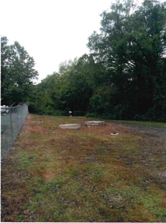
MH 1865 During Cleanup – 5/23/2024
