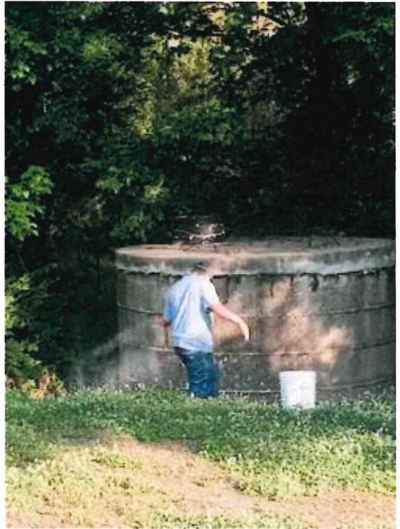
MH 1865 During Cleanup – Spreading Lime
