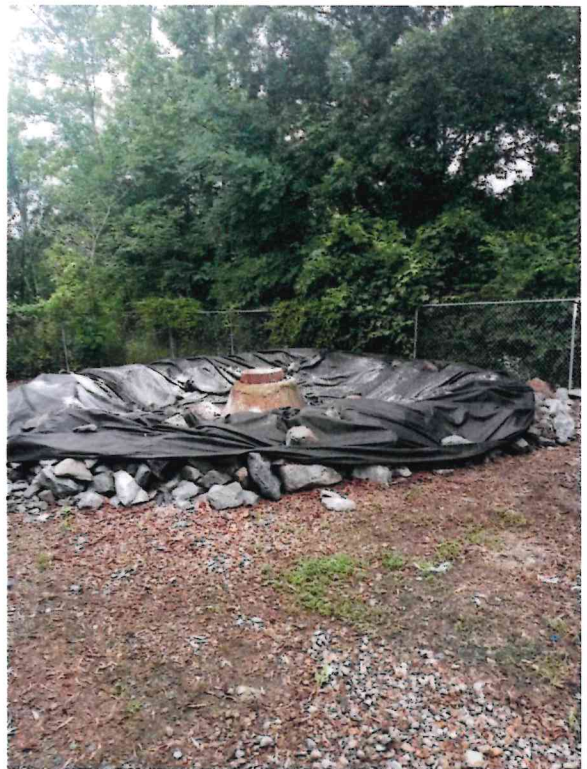
MH 1866 After Cleanup – 5/23/2024
