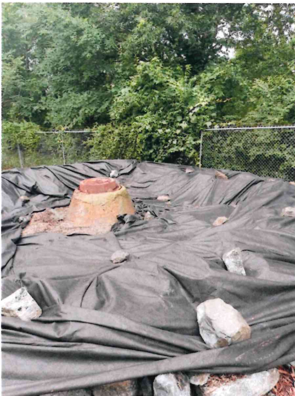
MH 1866 After Cleanup – 5/23/2024
